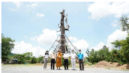
Fig. 11. The first project of lightning protection of a big tree in Thailand at Wat Prathom Wiwek
