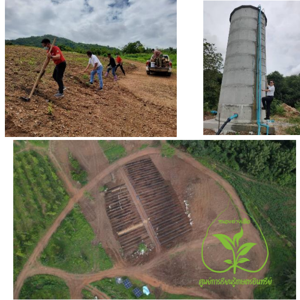
Fig. 7. Solar pump and water resource system with 27 cubic meter water storage for organic farming
